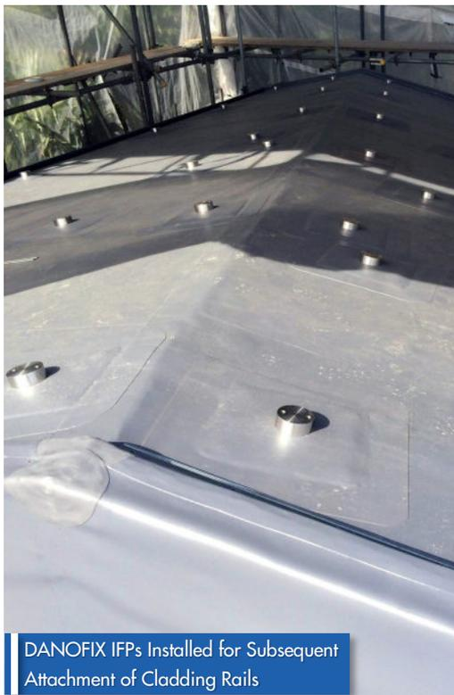
DANOFIX IFPs Installed for Subsequent Attachment of Cladding Rails
